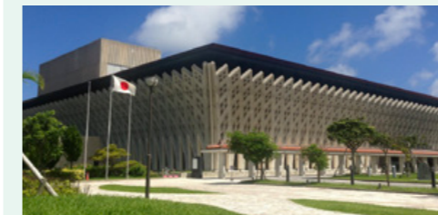
National Theater Okinawa (Primary contractor: Taisei Corporation; PS Construction Co., Ltd. was responsible for PCa production)
