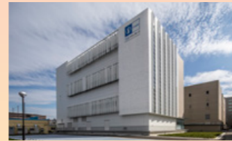
Chugai Pharma Manufacturing Co., Ltd. UK4: Bio-API Manufacturing Building UK4
