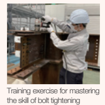
Training exercise for mastering the skill of bolt tightening
