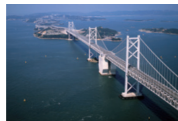
1985 Minami & Kita Bisan-Seto Bridges [substructure, North segment]
