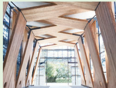
*2 Technology utilizing CLT: Inside of a wind tunnel test building (before wind tunnel installation)
