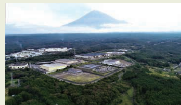
Fujisan Nanryo Industrial Park Development Project
